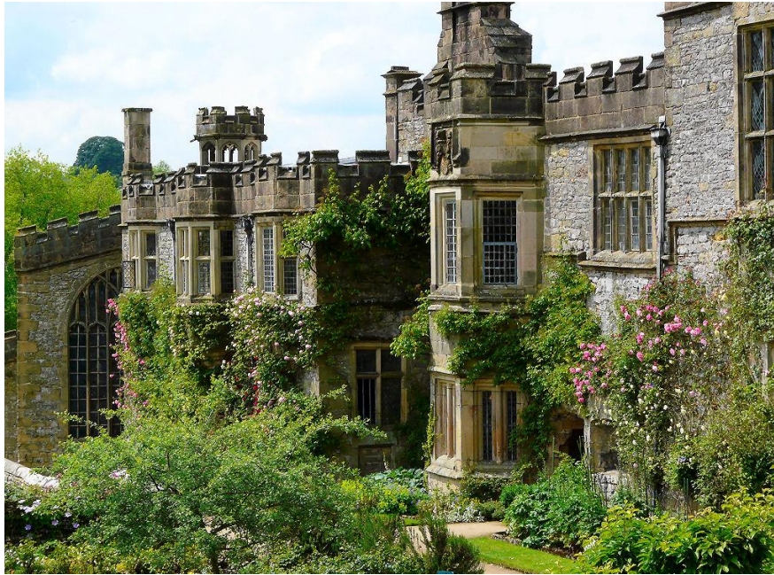
South front parapet, Haddon Hall, Bakewell (Derbyshire)
